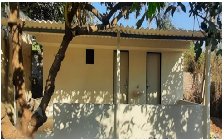
Renovation of toilet block
