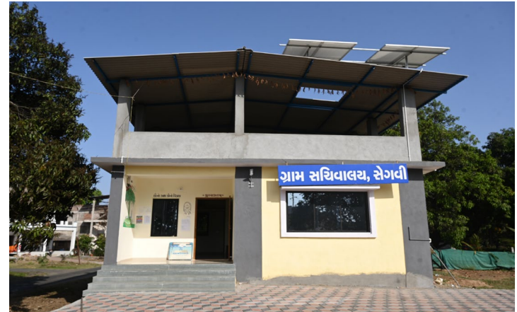
Renovation of community hall
