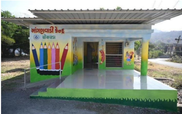
Renovation of anganwadi
